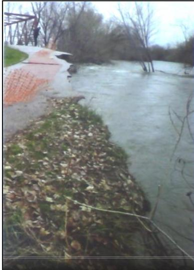
At the Sunroc gravel pit at the head of Eagle Island one of the pits started filling with water. If the pit wall gave way, the entire river could have diverted down the south channel, causing major flooding. To complicate matters, the West Boise Waste Water Treatment Plant lies directly downstream. The Army Corps of Engineers built 4400 feet of barrier, and Aire built a flood diversion water-filled tube. Muscle walls filled with water were also set up and a disaster was avoided.
